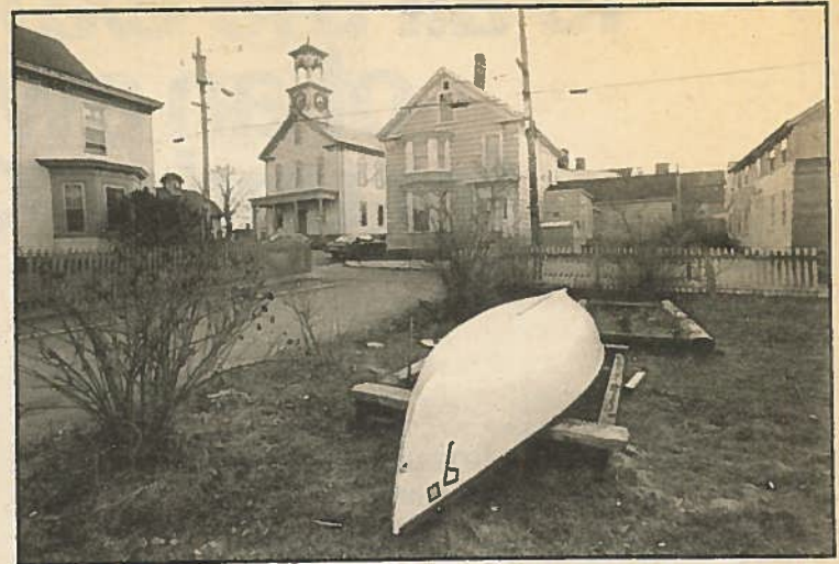
Puddle Dock: Most of the houses were either leveled or restored.
