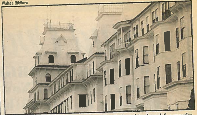
Wentworth-by-the-Sea: The New Castle hotel is closed for repairs.
